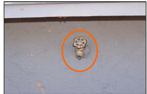
5. Slowly open the valve at the water meter. Don't just “jerk” the valve open. Open the valve a quarter turn every 5-10 seconds. This won't “shock” the plumbing lines possibly causing a leak within the system.
